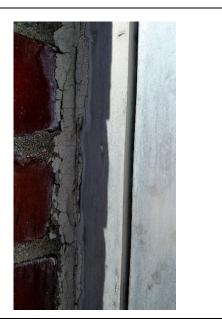
**Coating on interior concrete surfaces** were identified as containing less than 1% asbestos; however, it is recommended that this material be handled as an ACM. OSHA has issued several letters of interpretation with regard to materials that contain trace amounts (< 1%) of asbestos. The letters indicate that certain work practices are required for materials that contain asbestos in concentrations of <1%. The work practices specified by OSHA include:
